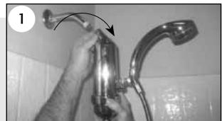
**CAUTION:** Threads from shower arm may cut Gasket if improperly installed. This may result in leakage around the Collar. If leak persists, use Teflon tape which is provided. Wrap Teflon tape around threads on existing shower arm 1 1/2 times. Re-thread Collar clockwise directly onto existing shower arm until tight. Do not over-tighten.
